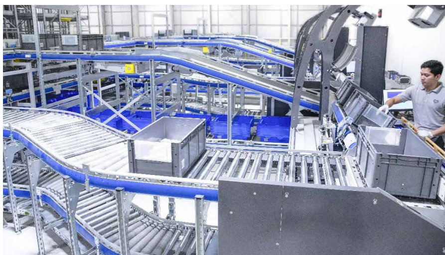
Al-Nahdi Distribution Centre (IMDAD) has a capacity of picking almost 100,000 order lines and over 5,500 shipping totes per day with the automated systems.
